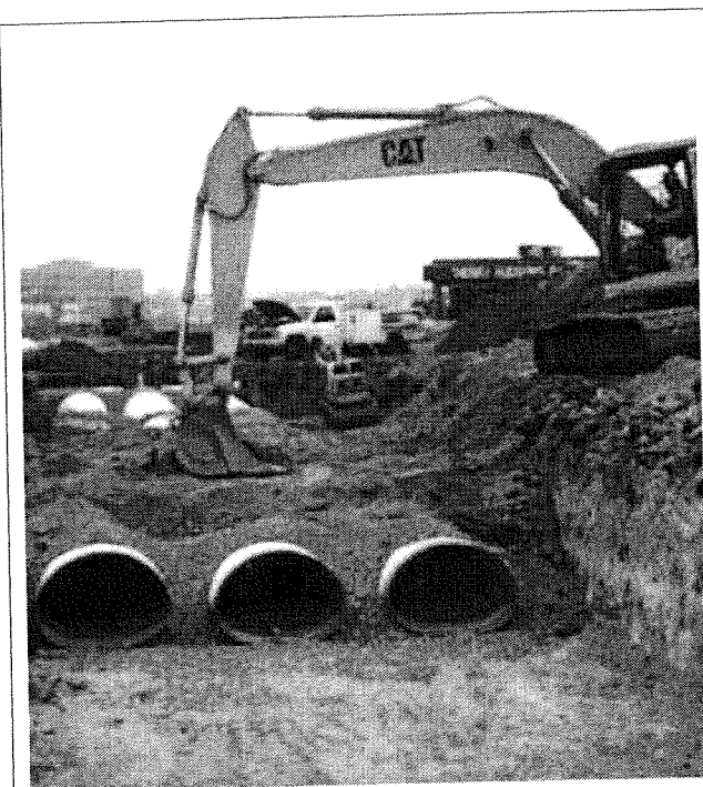
Pipe-arch for low profile application.
